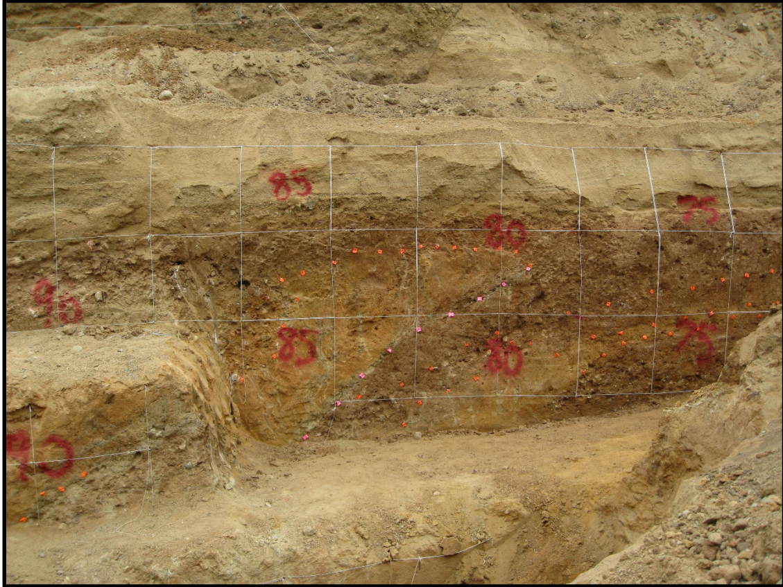
Figure 9 - View looking west at south dipping pre-Holocene bedding plane fault with a possible reverse sense of displacement in GDC's east trench. This trench was excavated across the southeastern portion of Site 2, and extends into Site 1; fault noted by pink flagging in the center of the photo. The upward termination of this fault, located right of Station 80 (about station 77), is within a fissure fill, which upon close inspection, is overlain by a mudflow deposit and soil, reported to be about 30 ka. In this photo, the Pleistocene age older alluvium (debris flow deposits) are overlain by a thin mudflow deposit, overlain by sands of the Argyle Channel.
